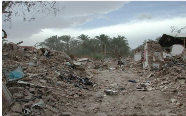
Road blockages caused by debris from roadside structures
